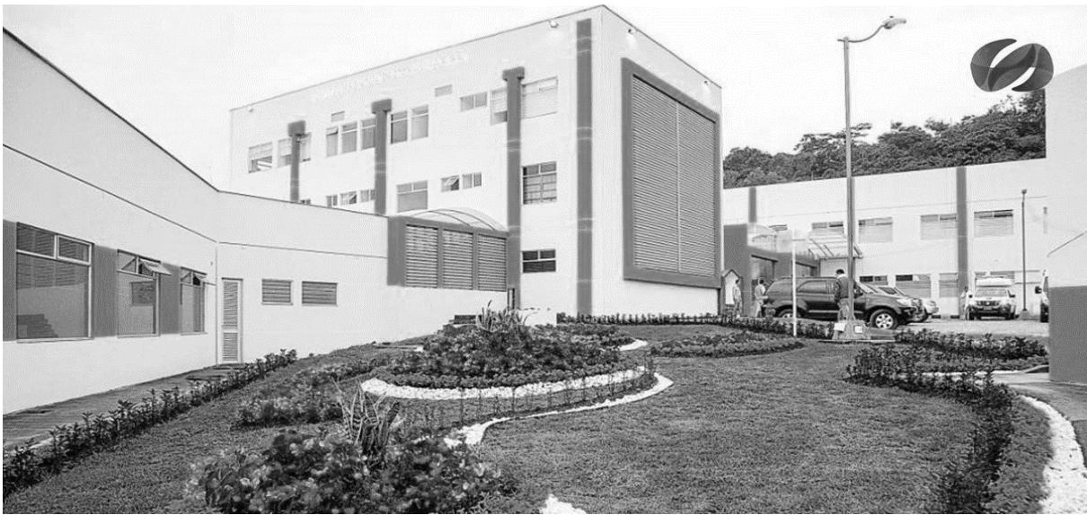
Infraestructura Hospital Regional de Moniquita E.S.E.
